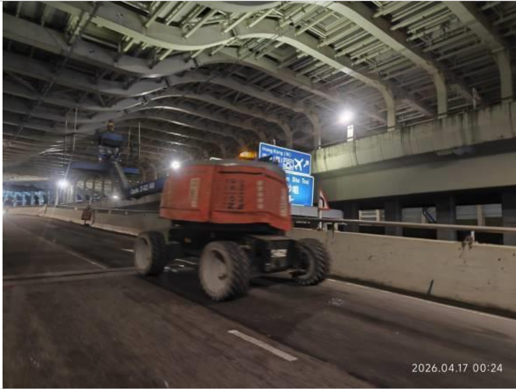
Mitigation measure implemented for Cherry picker on site
